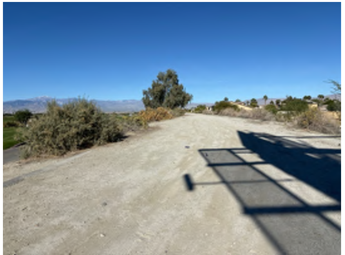
Photo 2: View of east levee top.
