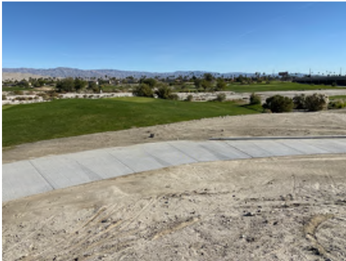
Photo 7: View of golf course and general site conditions from Whitewater river west levee top.
