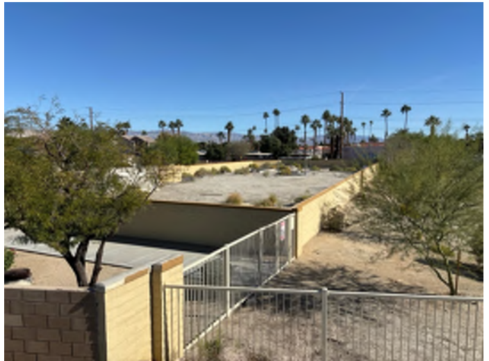
Photo 4: View of Coachella Valley Water District facility.
